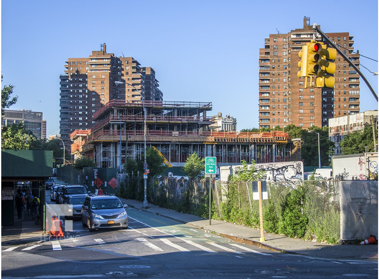
145 Clinton Street. Park will be located at right. Photo by Tectonic
