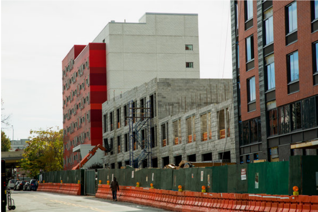
Construction at the Navy Green housing complex. Pablo Enriquez for The New York Times
