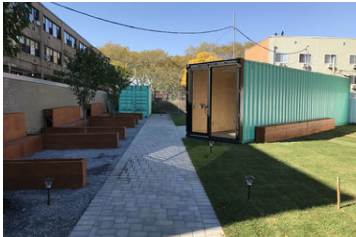
A youth and community clubhouse made from re-designed shipping containers takes over a vacant lot on Chester Street and Dumont Avenue in Brownsville and debuts on Oct. 19.
