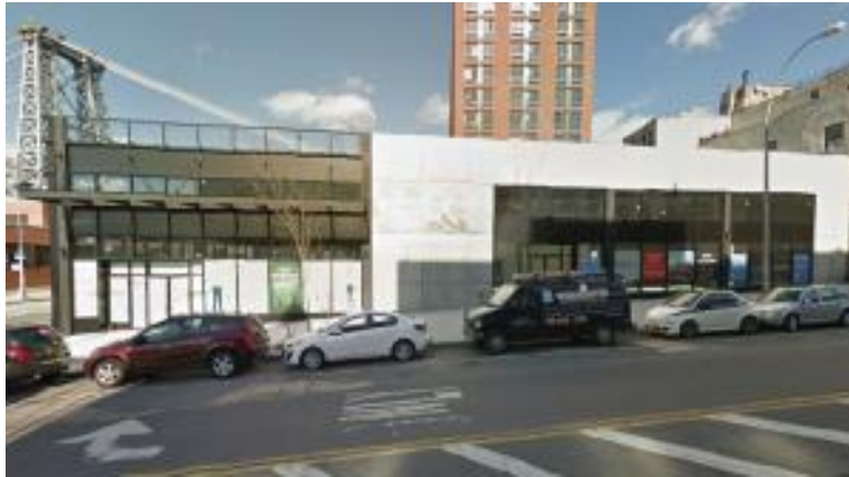
11 Broadway in South Williamsburg.
