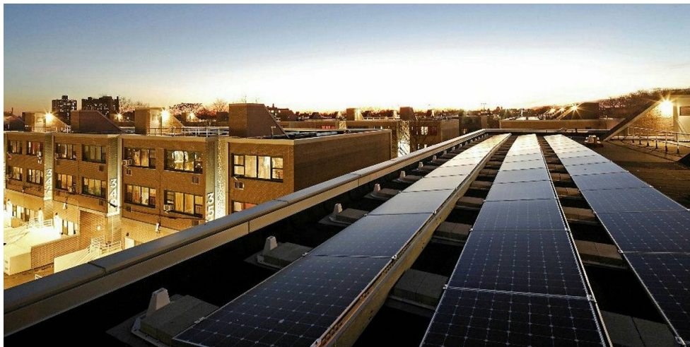
Brooklyn's Marcus Garvey Apartments generate and store electricity on-site while offering demand-response services to utility Con Ed. Photo: Enel X
