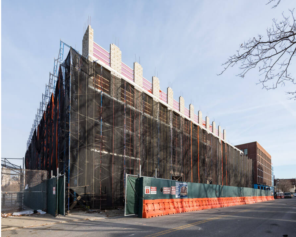
5 Blue Slip under construction in March 2016. Photo by Field Condition
